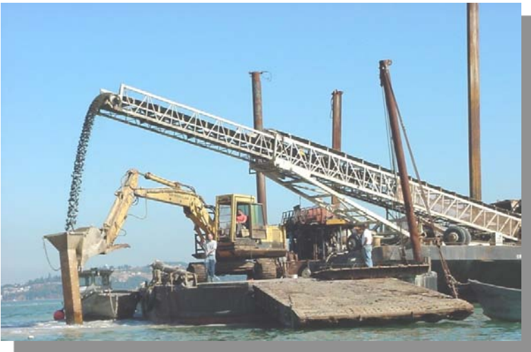
Cap Placement Using Tremie and Conveyor
