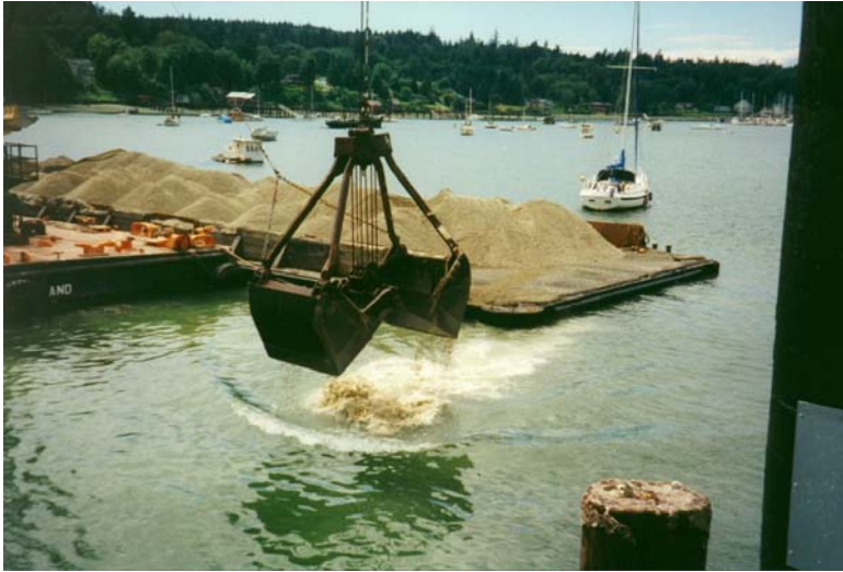
Cap Placement Using Bucket
