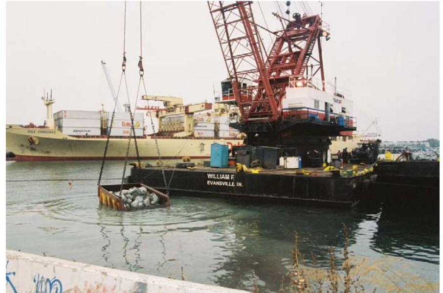
Armor Rock Placement with Skip Box
