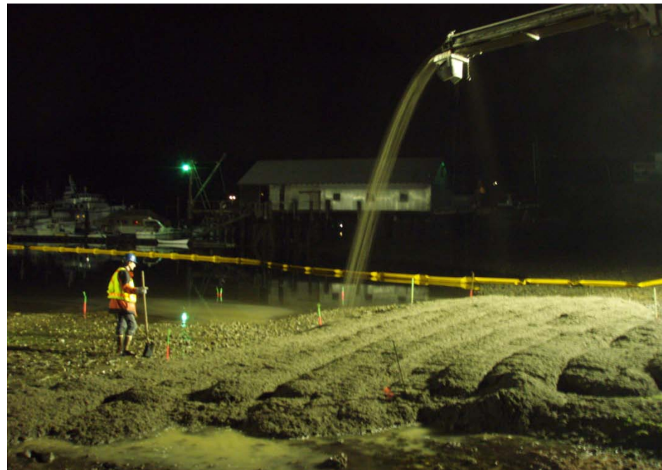
Conveyor Placement of Thin Layer Cap
