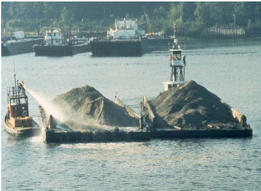
Hydraulic Spray Placement at Eagle Harbor, Washington
